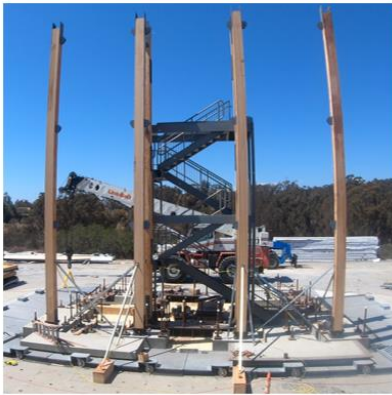
Left: Columns, stairs and temporary bracing; Middle: Level 1 beams and slabs; Right: Installation of Level 1 safety rails.
