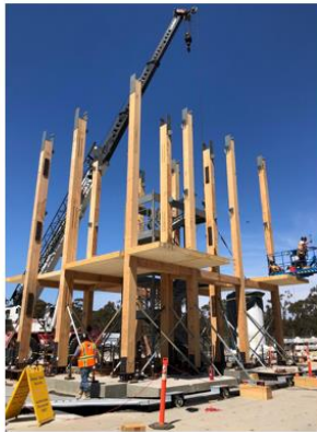
Left: Columns, stairs and temporary bracing; Middle: Level 1 beams and slabs; Right: Installation of Level 1 safety rails.
